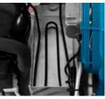
Evaporation at zero cost The water produced by defrosting evaporates by exploiting the heat dissipated by the refrigeration system.
